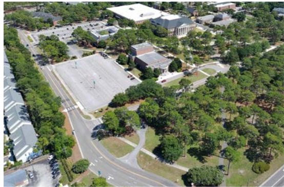
Existing Bird's Eye Aerial
