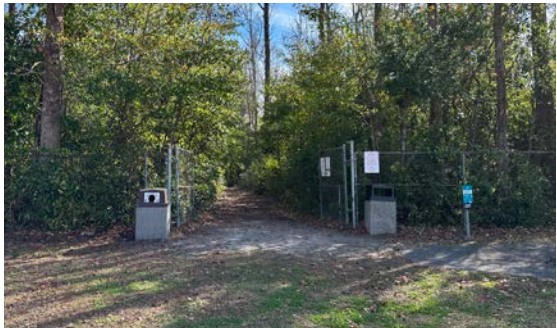
Existing Entry Point and Perimeter Fencing
